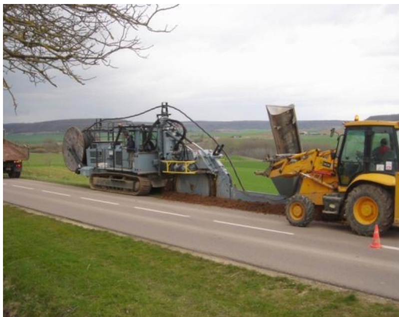
Figure 5 Trancheuse et raccordement
